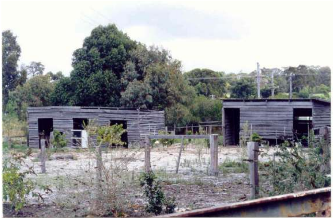
The stables next to Willyung Cottage. (not original) (Heritage TODAY 1999)
