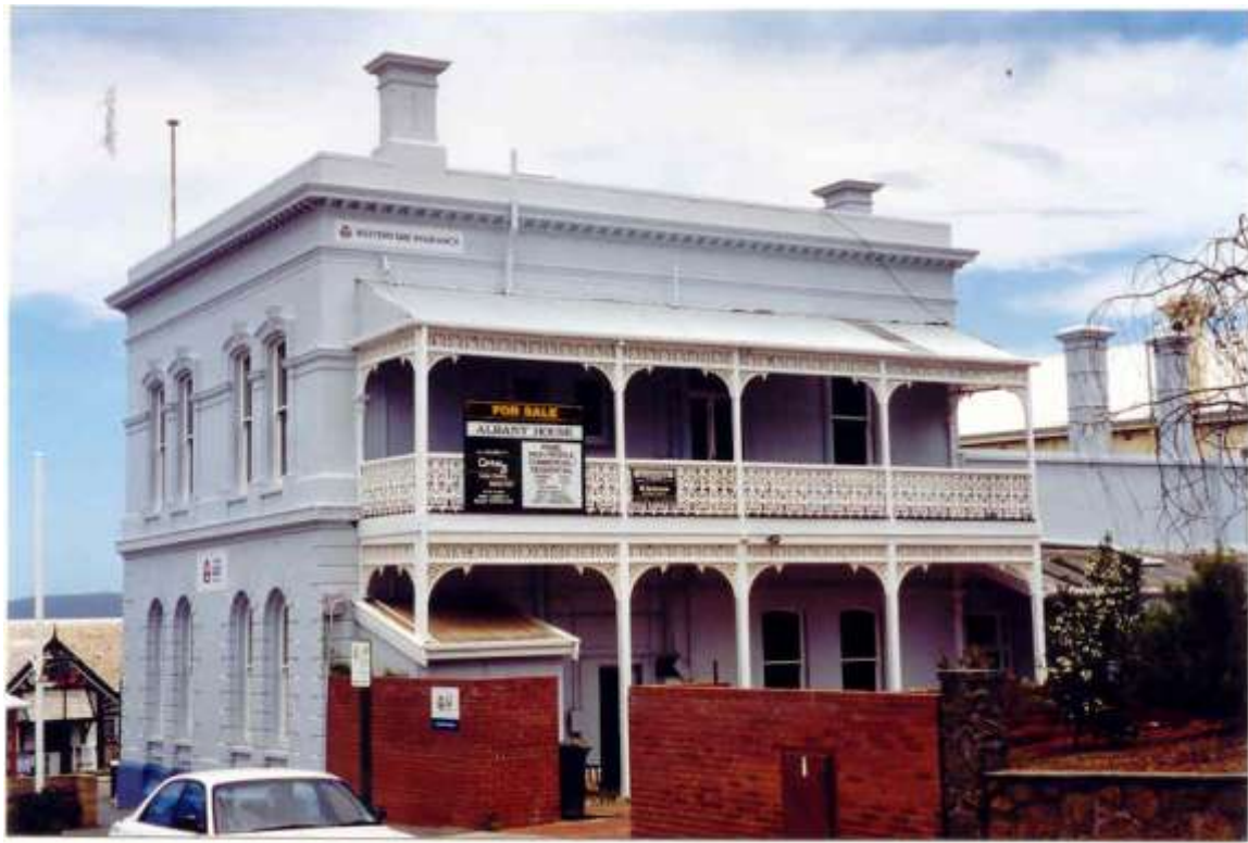
Albany House, rear view (Heritage TODAY, 1999)
