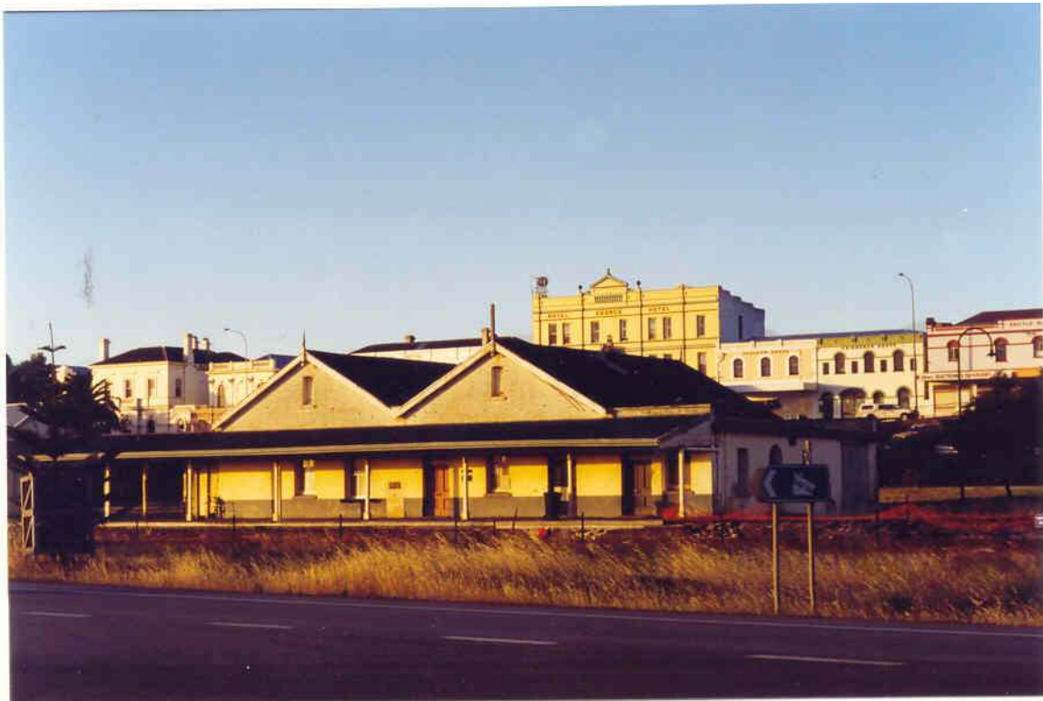
A rear view of the former warehouse looking up to Stirling Terrace.
