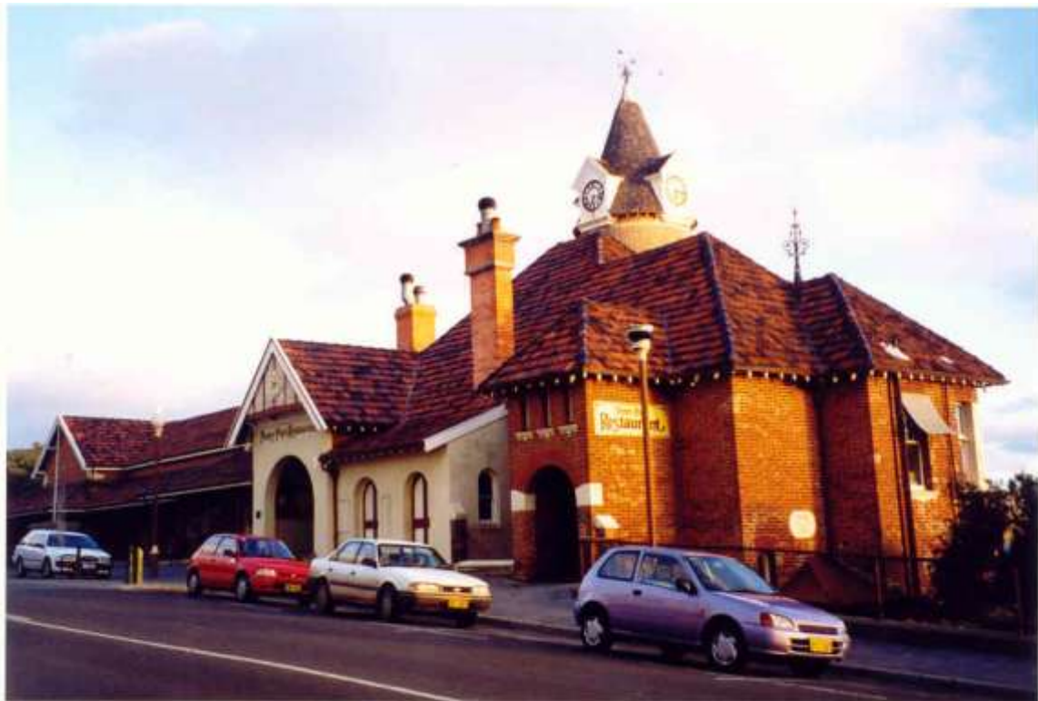
Old Post Office, View from Stirling Terrace. (Heritage TODAY, 1999)
