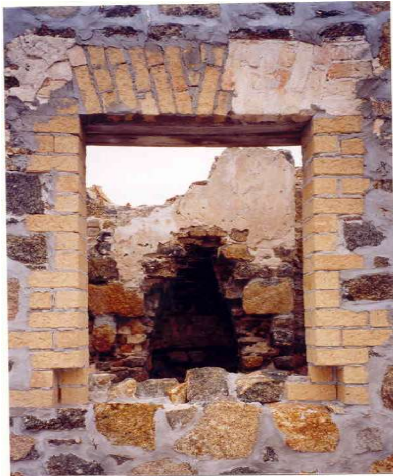
Lighthouse Keepers Cottage. (Heritage TODAY 1999)
