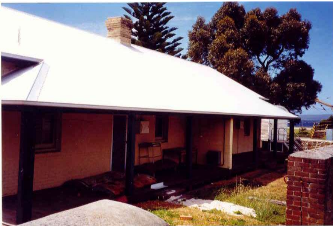
Former Police Quarters Heritage TODAY , 1999.
