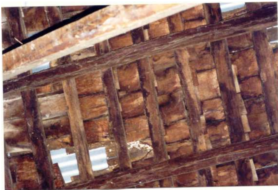
Internal view - wooden shingles under corrugated iron roof.
