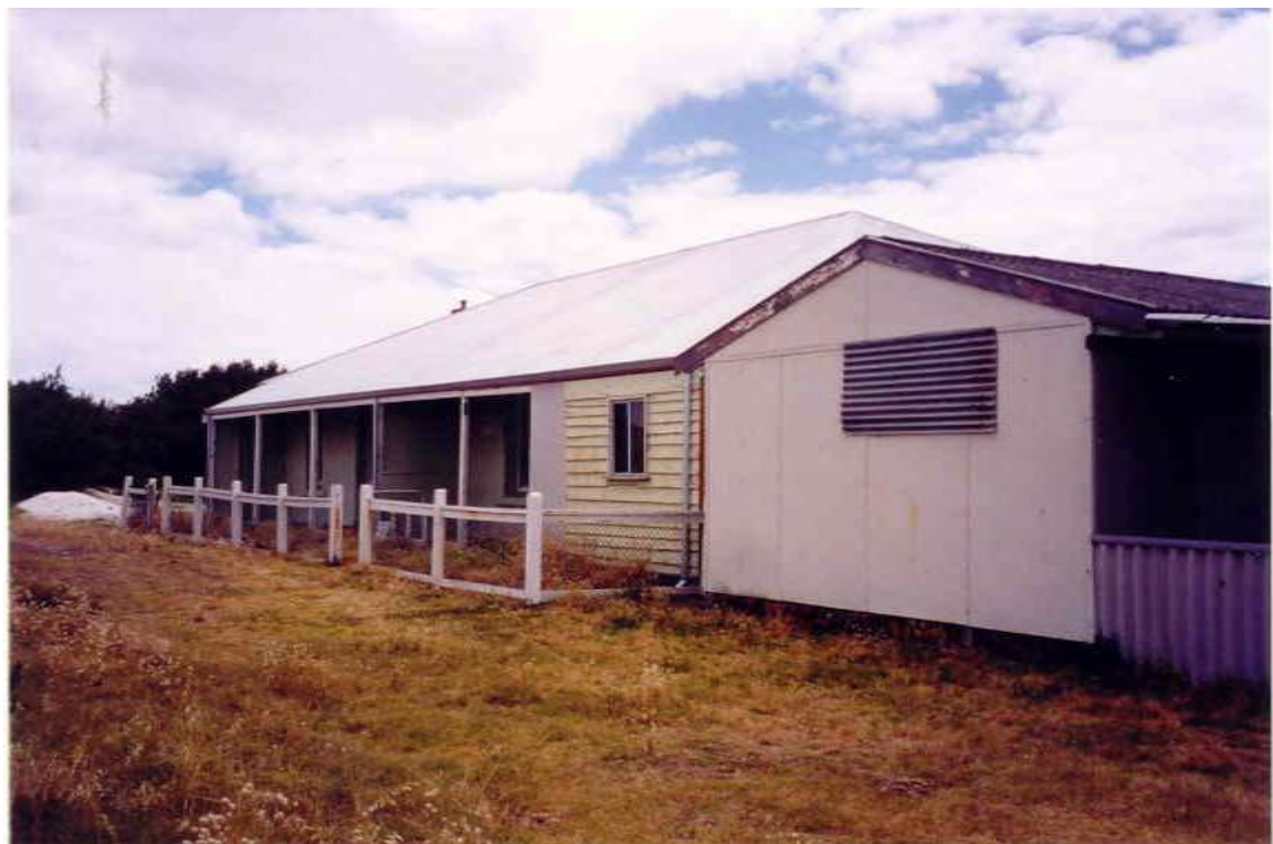
Pilot Station, front view, facing the ocean. Heritage TODAY, 1999.
