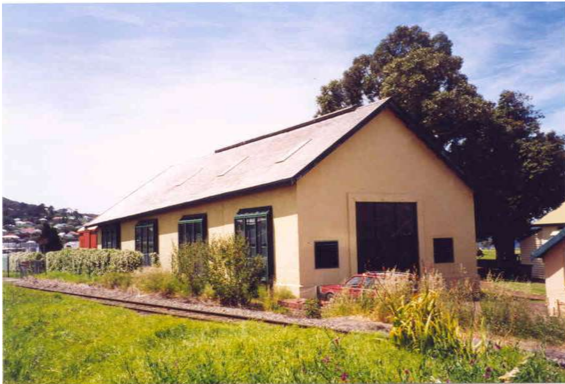
Former Police Quarters Heritage TODAY , 1999.
