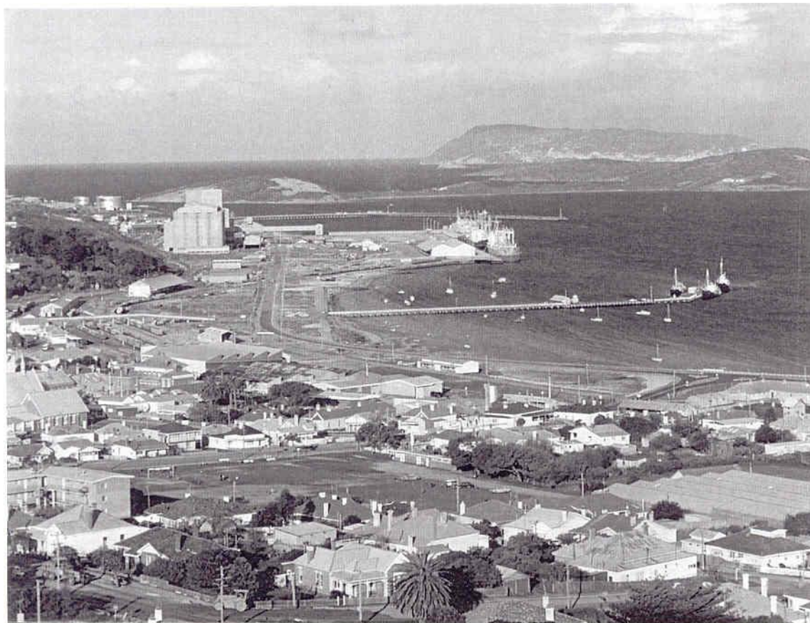
Photograph 45: View of Town of Albany and Princess Royal Harbour after the construction of the land backed wharves (Courtesy of the City of Albany Local Studies Collection)
