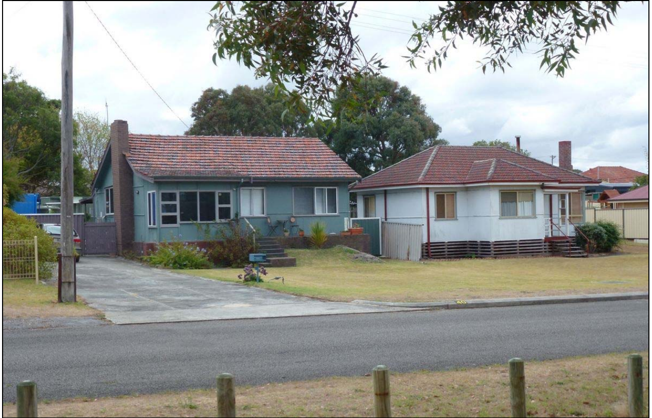
Photo 16: Fibro cottages in Burville Street.
