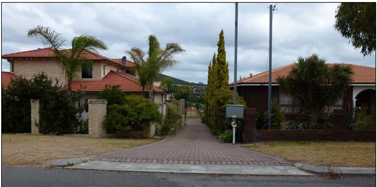
Photo 13: Redeveloped brick & tile housing on Hillman Street.
