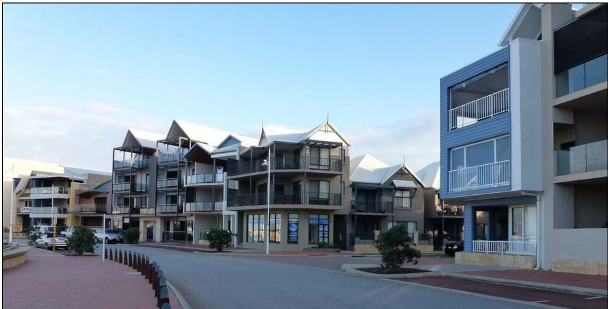
3 & 4 storey apartments with commercial use at ground level
