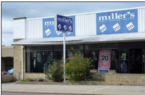
Freestanding sign inappropriate to town centre.
