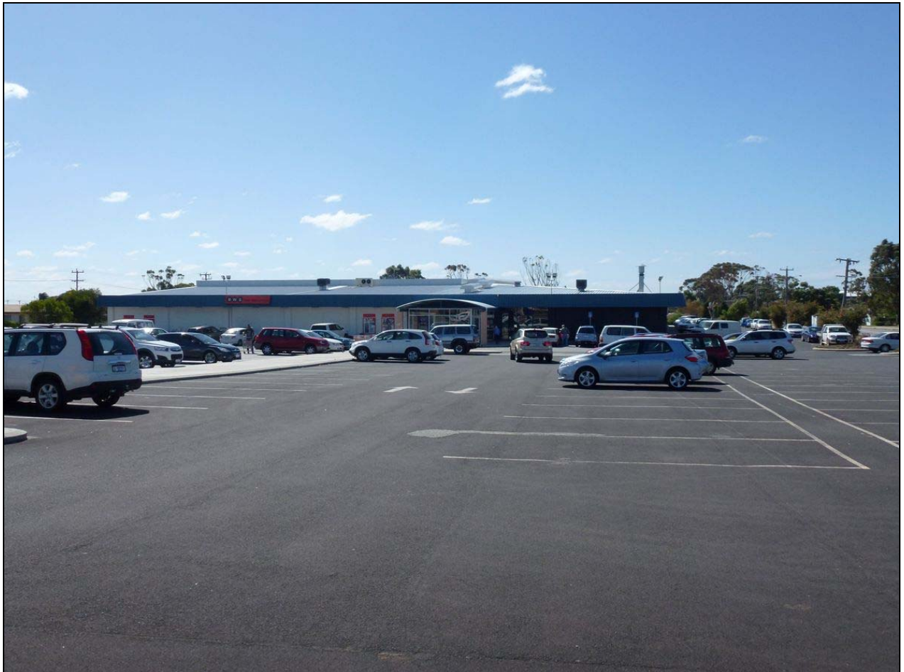
Photo 1: Spencer Park Shopping Centre
