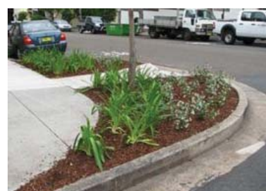
Typical crossing point where planting is used to direct traffic
