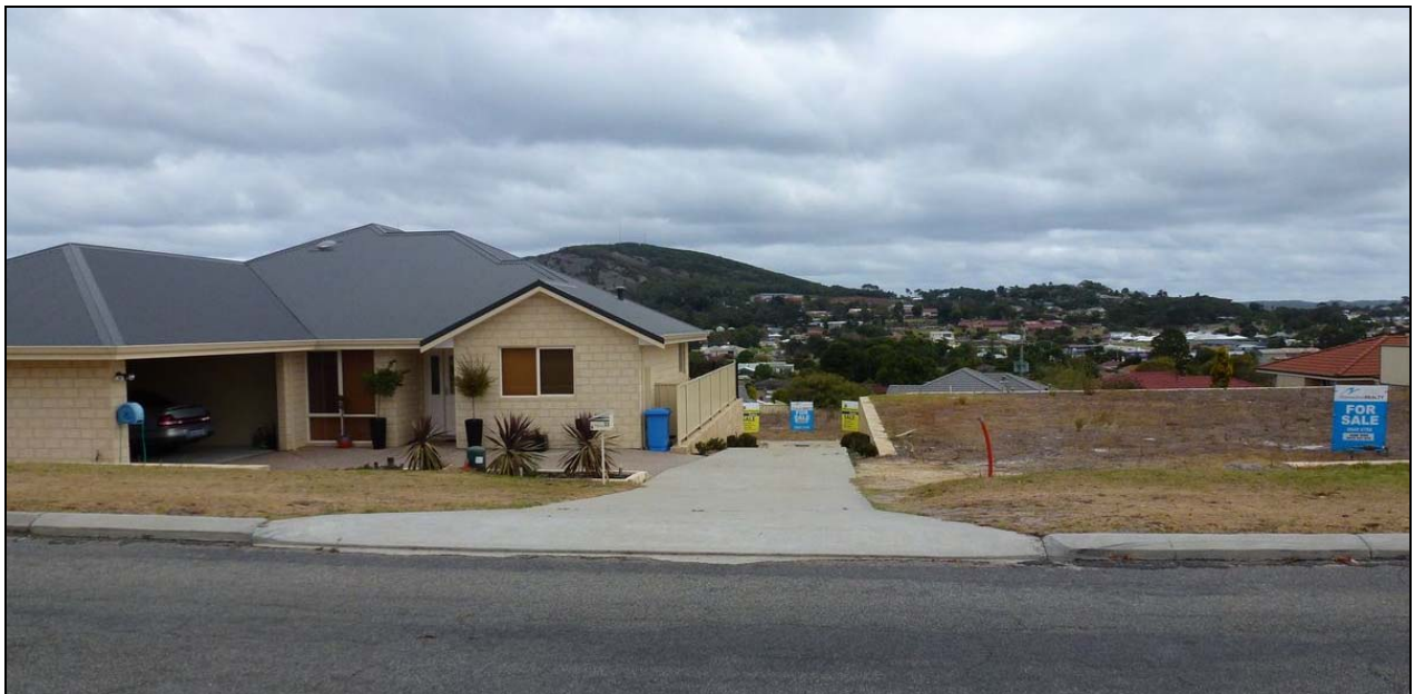
Photo 12: New Housing on Hillman Street together with recent battleaxe subdivision.
