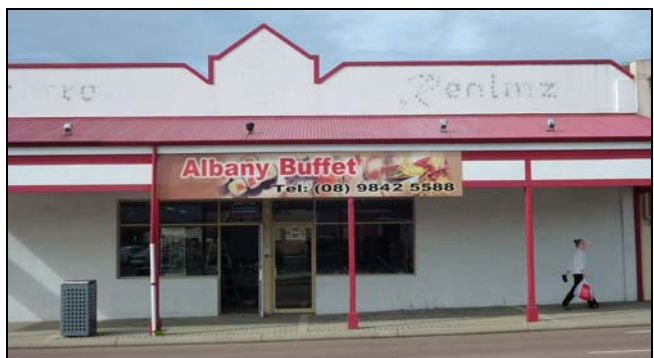
Sign design unrelated to fascia of awning.
