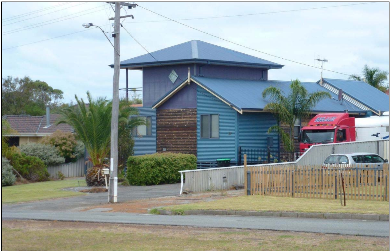
Photo 15: Renovated housing on Mokare Road.
