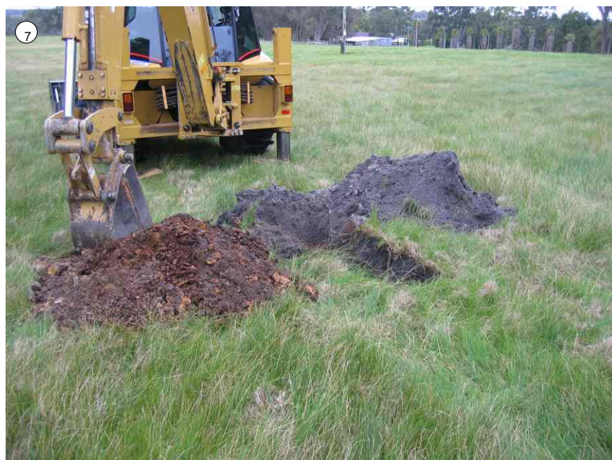
Grey sand over weak organo ferricrete over yellow silt in Sand over Silty Clay in the central east.
