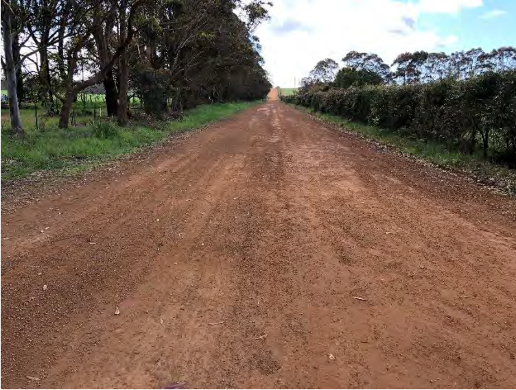
Figure 2.5 – Terry Road – Looking East
