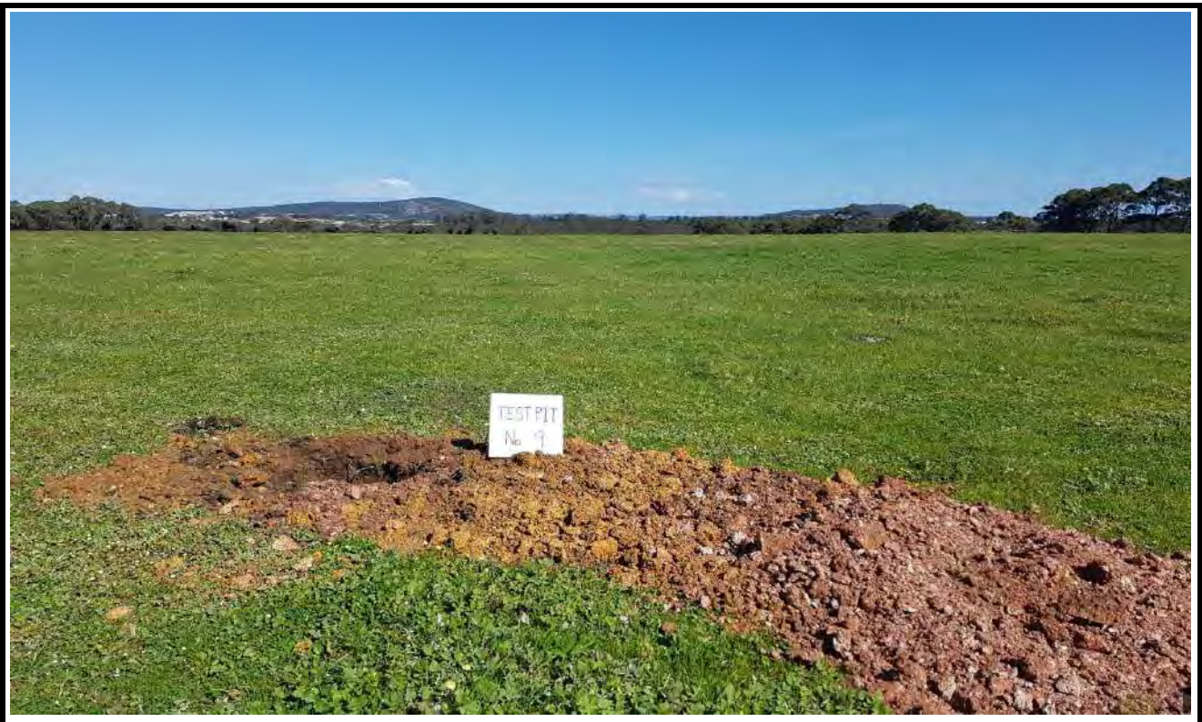
Test Pit No. 9 Spoil
