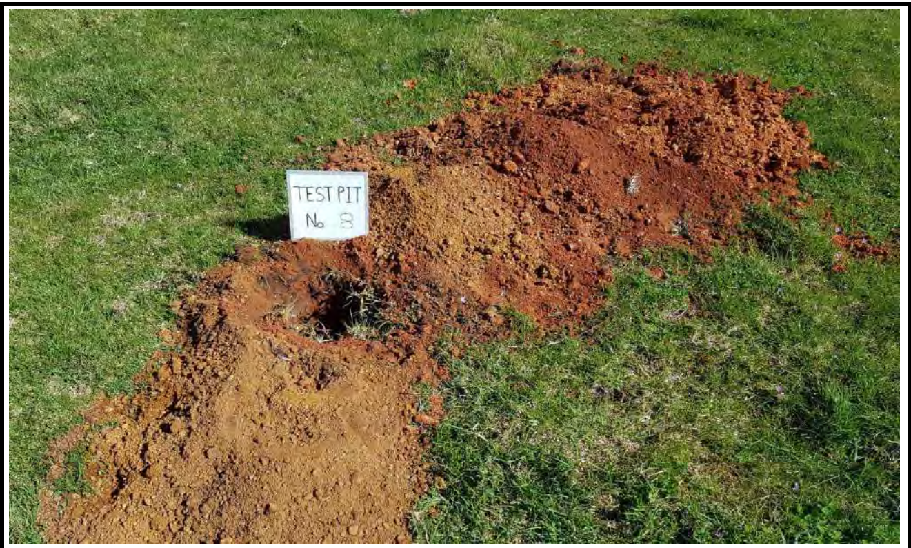
Test Pit No. 8 Spoil
