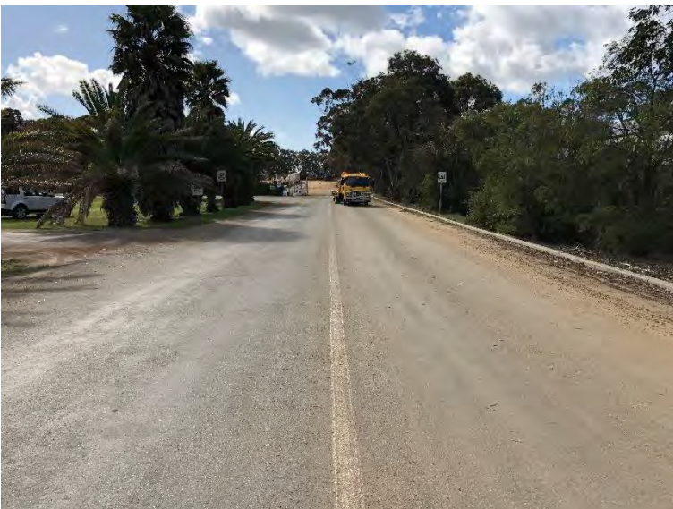
Figure 2.6 – Private Access Road – Looking East
