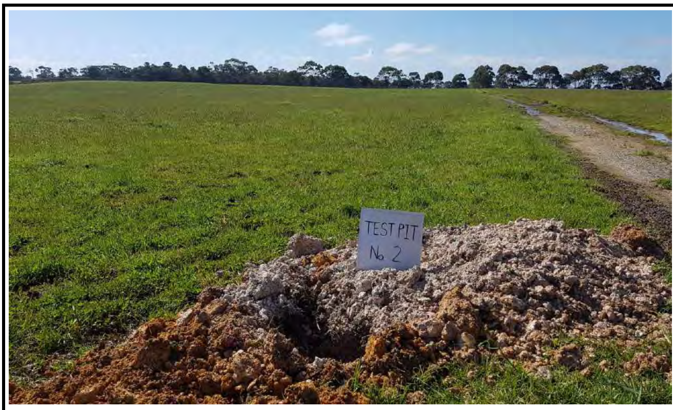
Test Pit No. 2 Excavation
