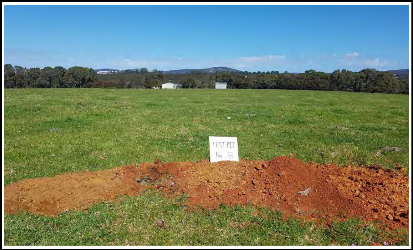
Test Pit No. 8 Excavation
