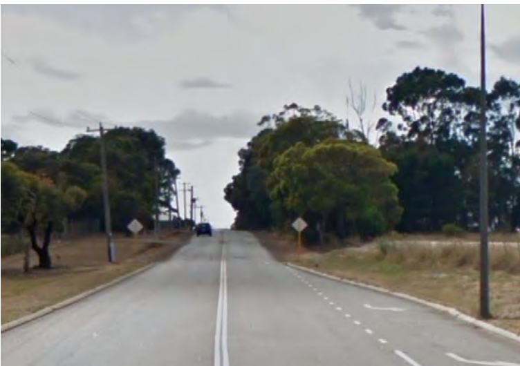
Figure 2.4 – Mercer Road – Looking East
