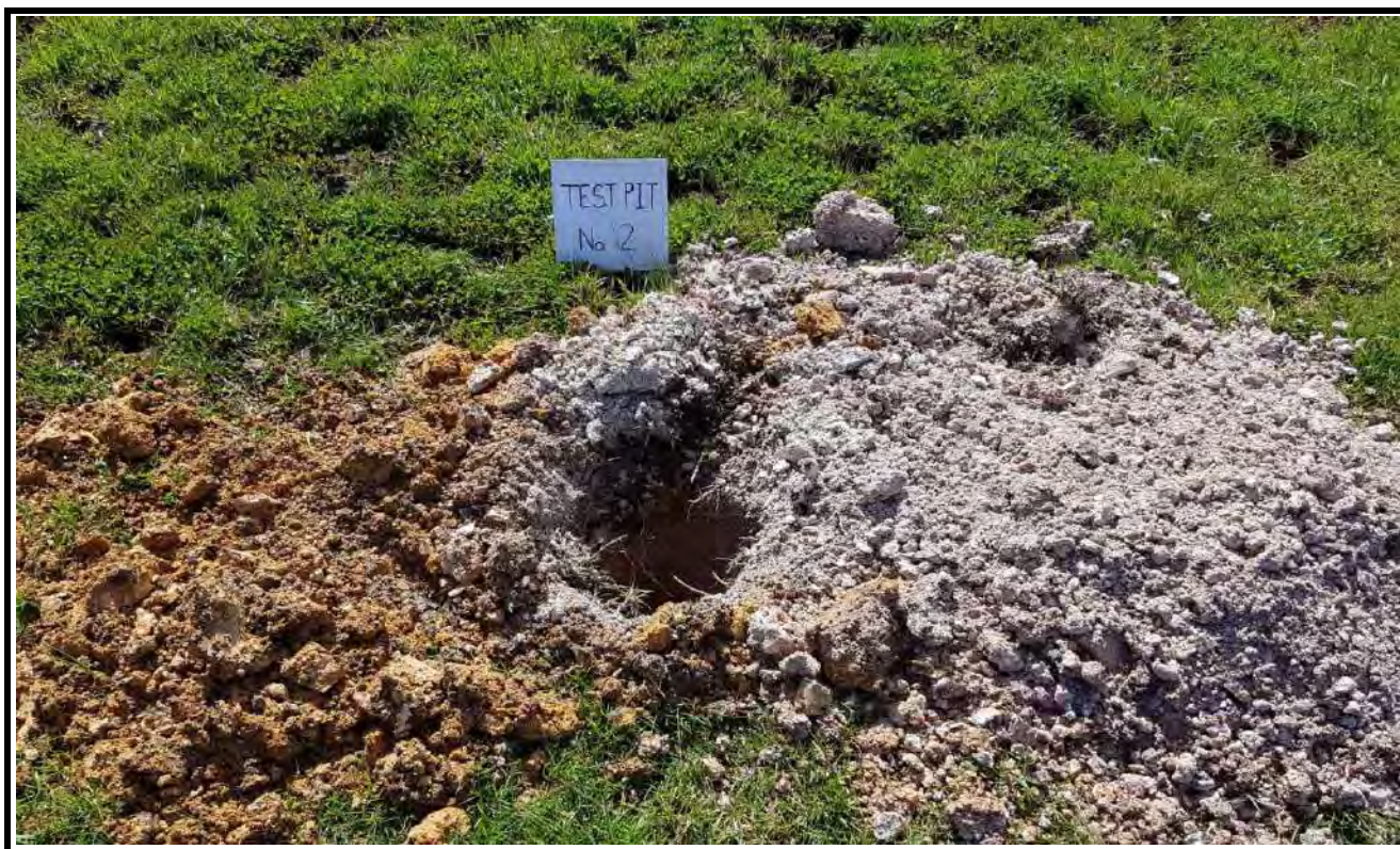
Test Pit No. 2 Spoil
