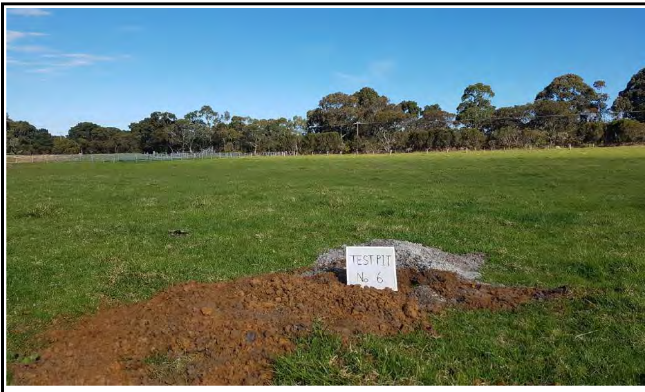
Test Pit No. 6 Excavation
