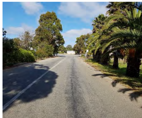
View from the Ardess Industrial Estate access way towards Chester Pass Road
