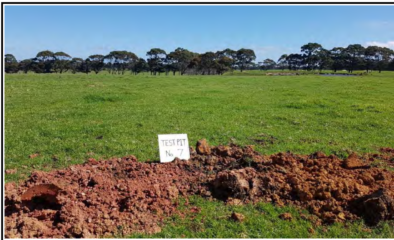
Test Pit No. 7 Excavation
