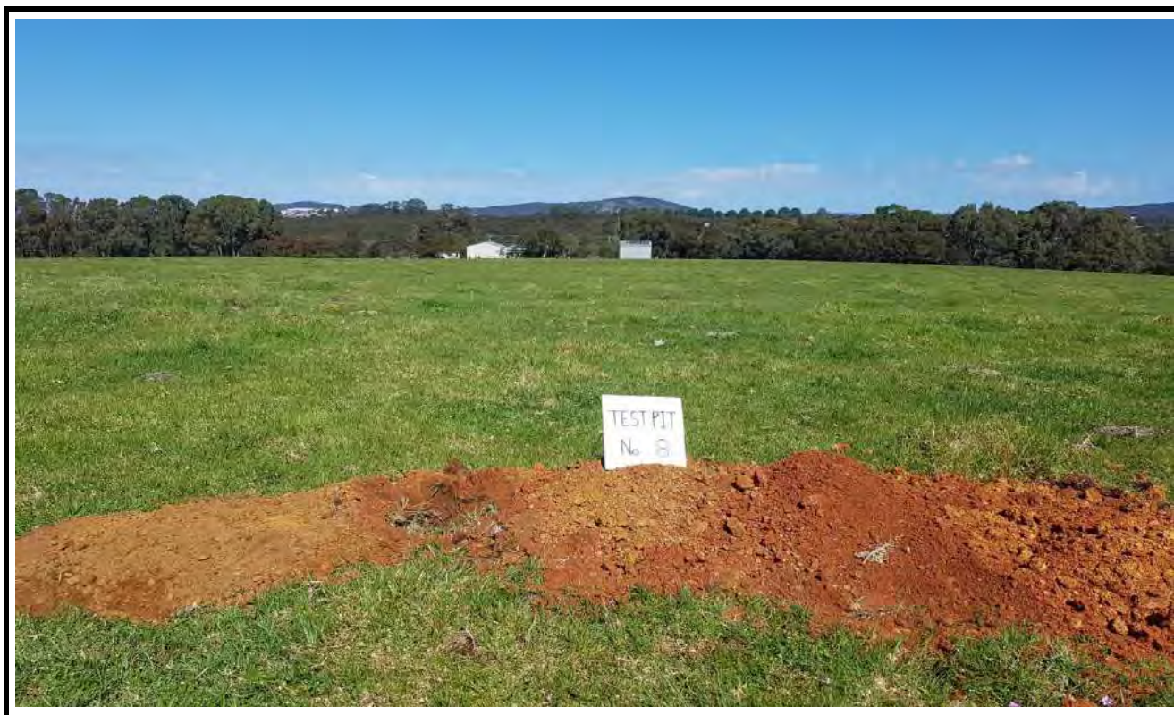
Test Pit No. 8 Excavation
