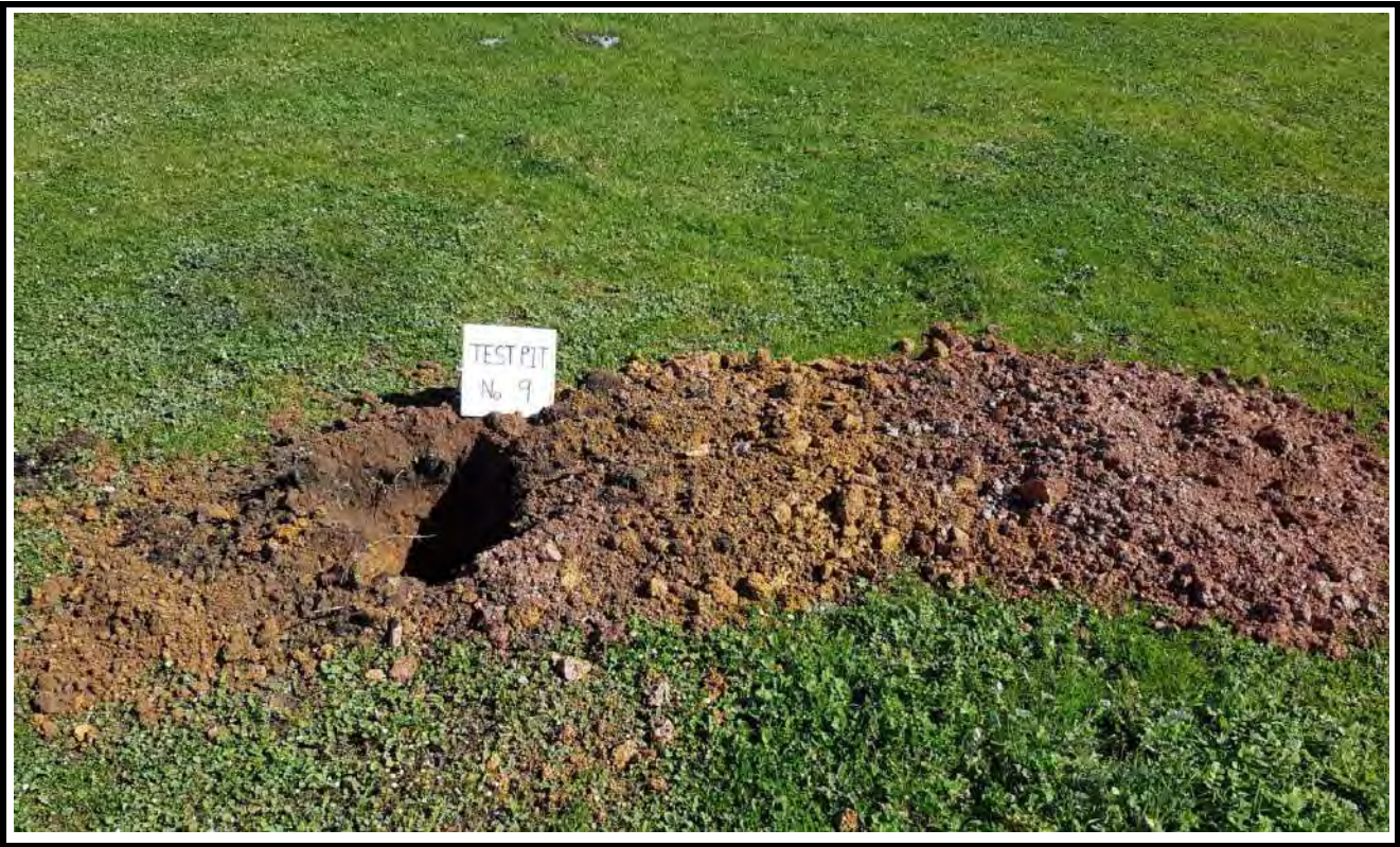
Test Pit No. 9 Excavation
