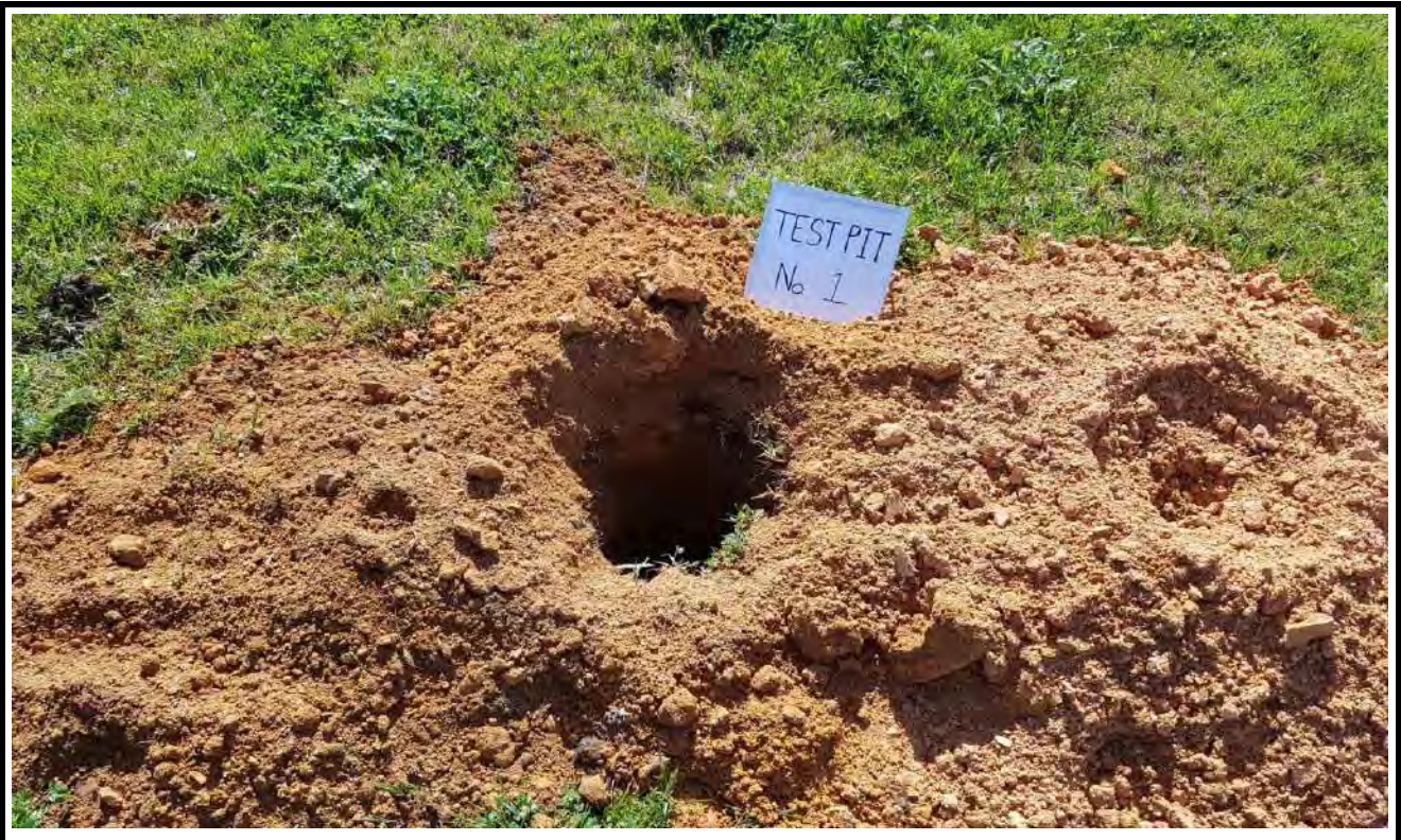
Test Pit No. 1 Spoil
