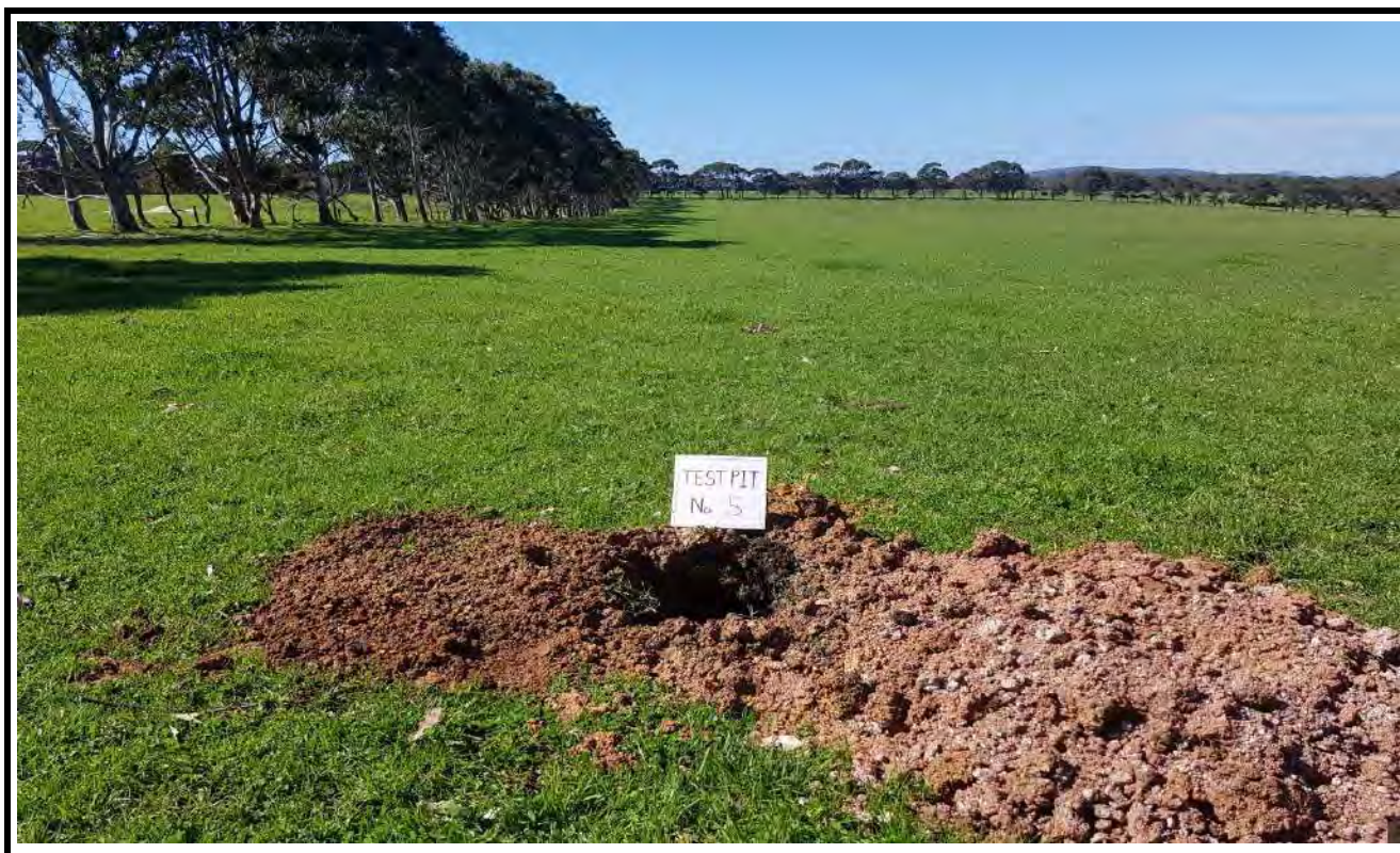
Test Pit No. 5 Excavation
