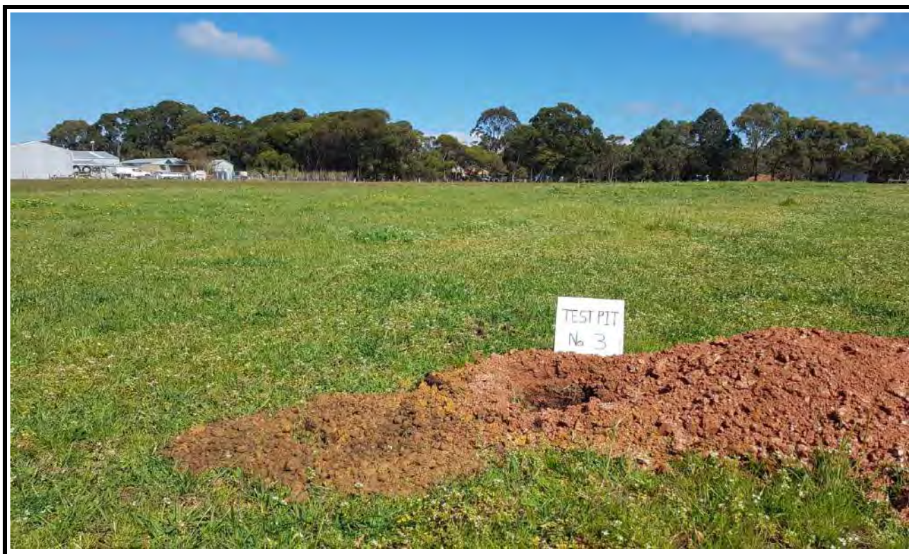
Test Pit No. 3 Excavation
