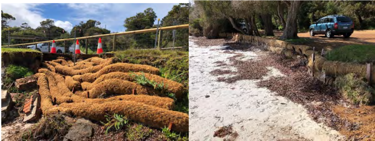
Figure 3.13 Coir Logs Installed by the City of Albany in 2021 to Combat Erosion
