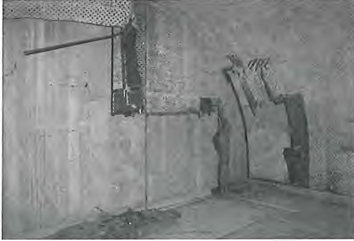
Engine Room [City of Albany, 2010]
