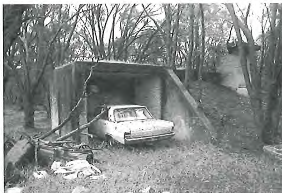
Garage [City of Albany, 2010]
