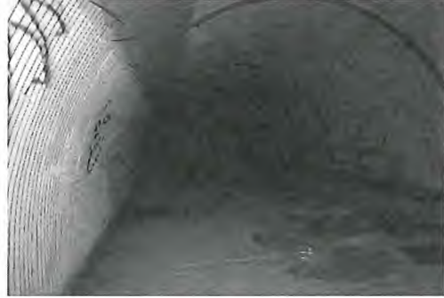
Tunnel/bunker [City of Albany, 2010]
