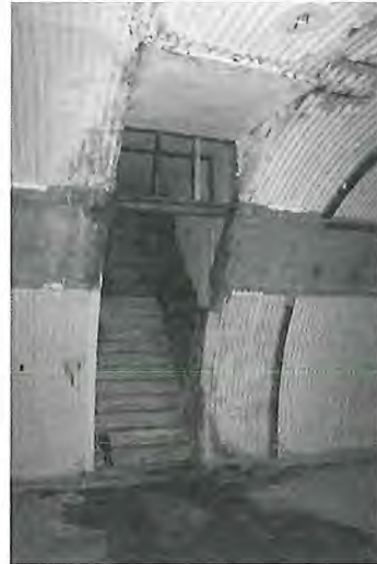
Stair to tunnel/bunker [City of Albany, 2010]
