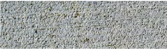
Name: Natural Grey Concrete Path Finish: Broomed
