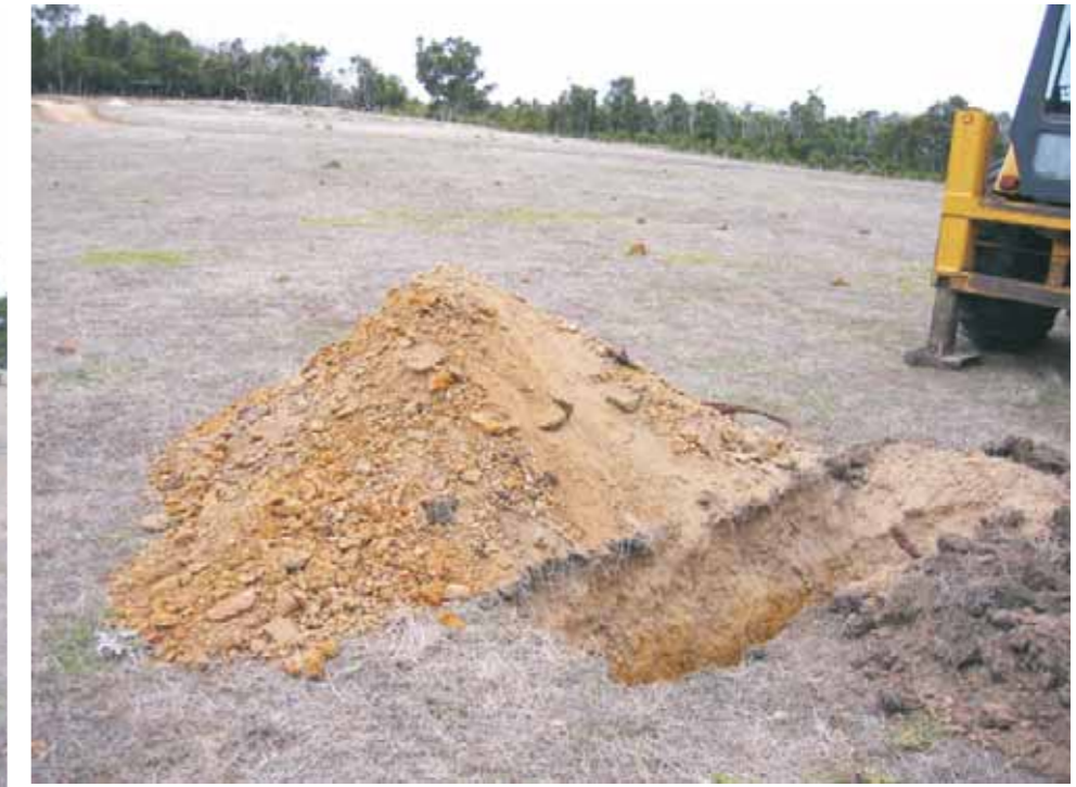
Soil test hole 5, looking towards the rocky soils
